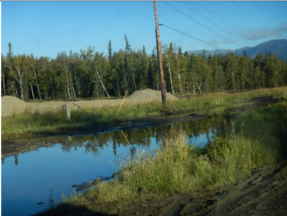
Ponding at corner of Trunk Road and Palmer-Fishhook Road.
