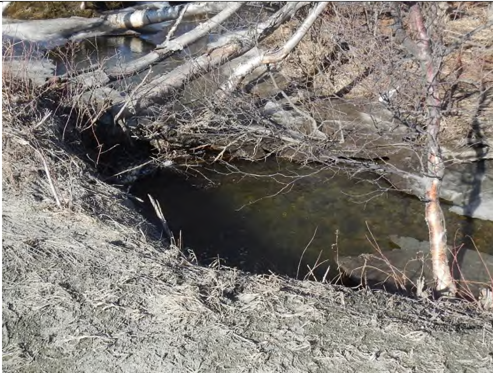
Sediment contamination at Wasilla Creek and Stringfield Road encroachment.
