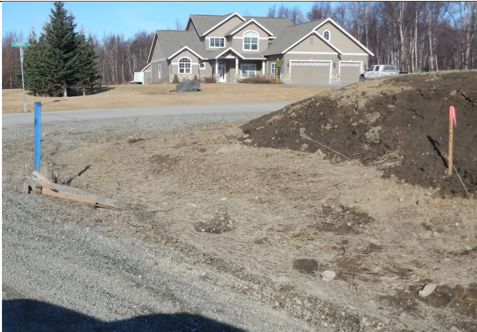
Corner of Commons and Tributary Avenue – looking west. Residential storage of large amount of material without BMPs near culvert.
