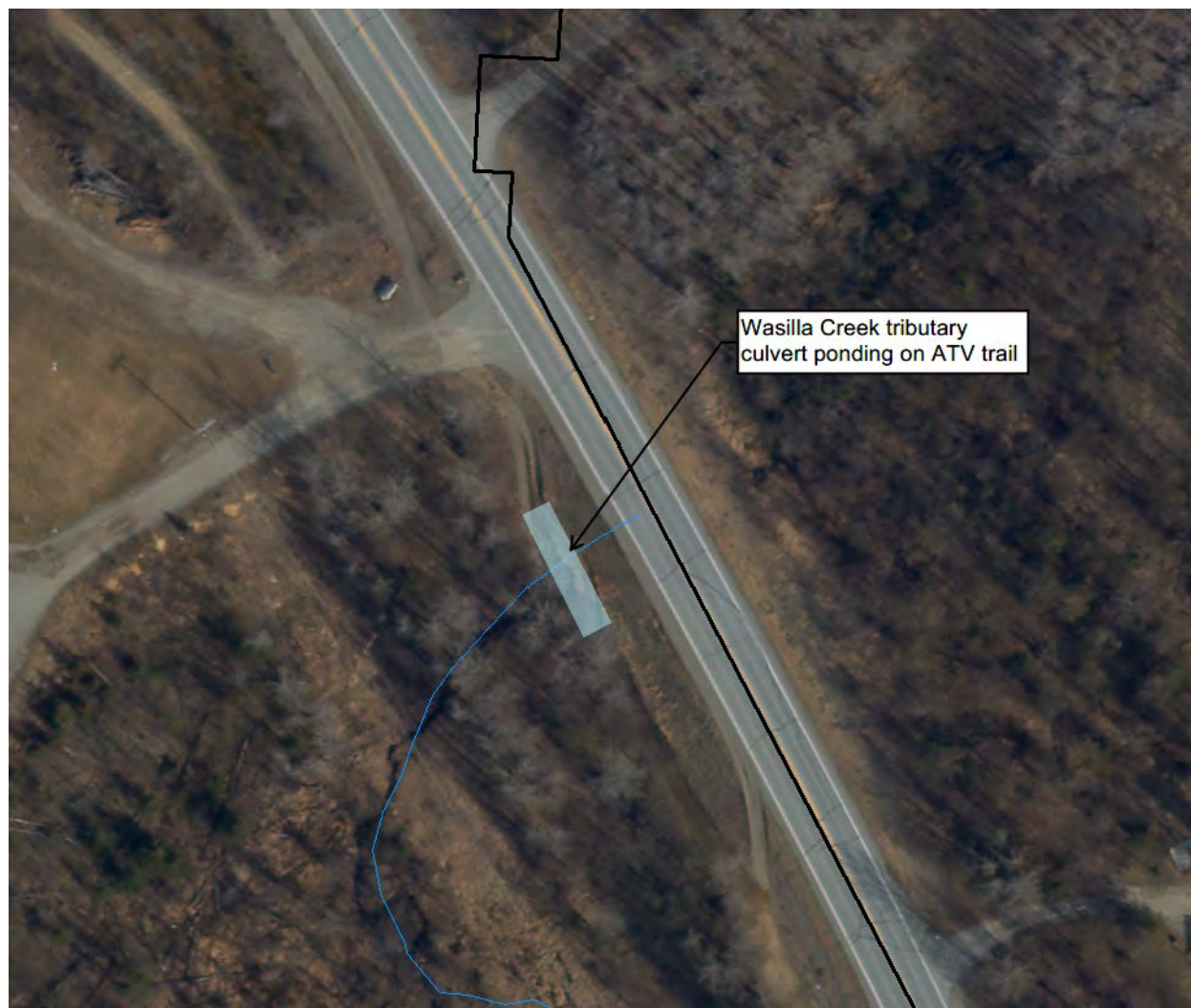
Figure 8: Wasilla Creek tributary culvert ponding on ATV trail at Palmer-Fishhook Road
