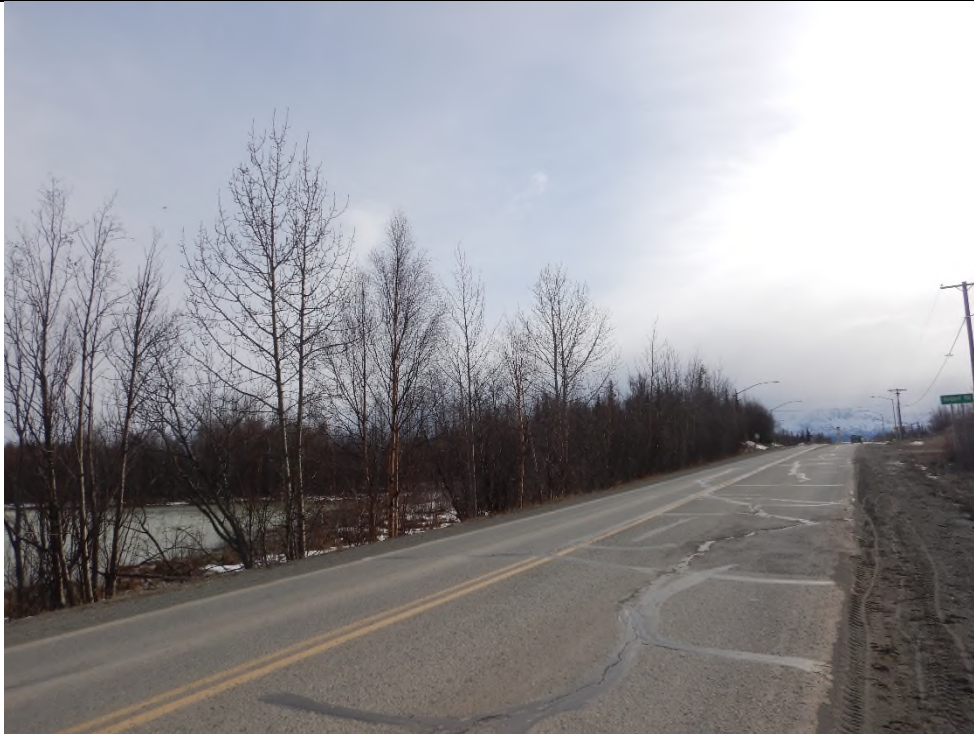
Shallow ditches along North 49th State Street.
