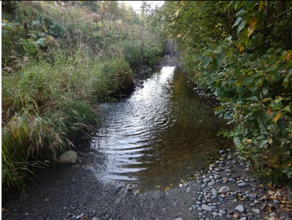
Wasilla Creek Tributary at Palmer-Fishhook Road undersized structure. Stream outfall on ATV trail at outlet.
