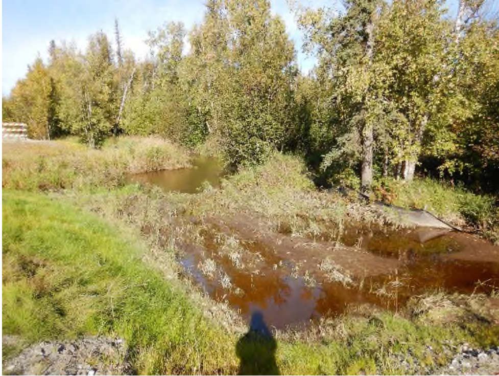
Ineffective BMPs at Nelson Drive.
