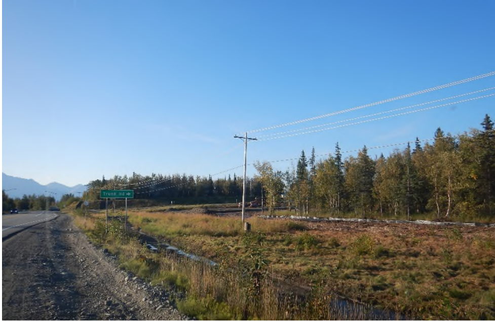
Ponding at corner of Trunk Road and Palmer-Fishhook Road.
