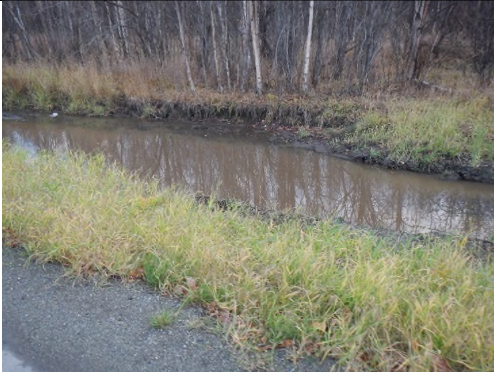
Ponding in ditches/ATV trails along Stringfield Road.
