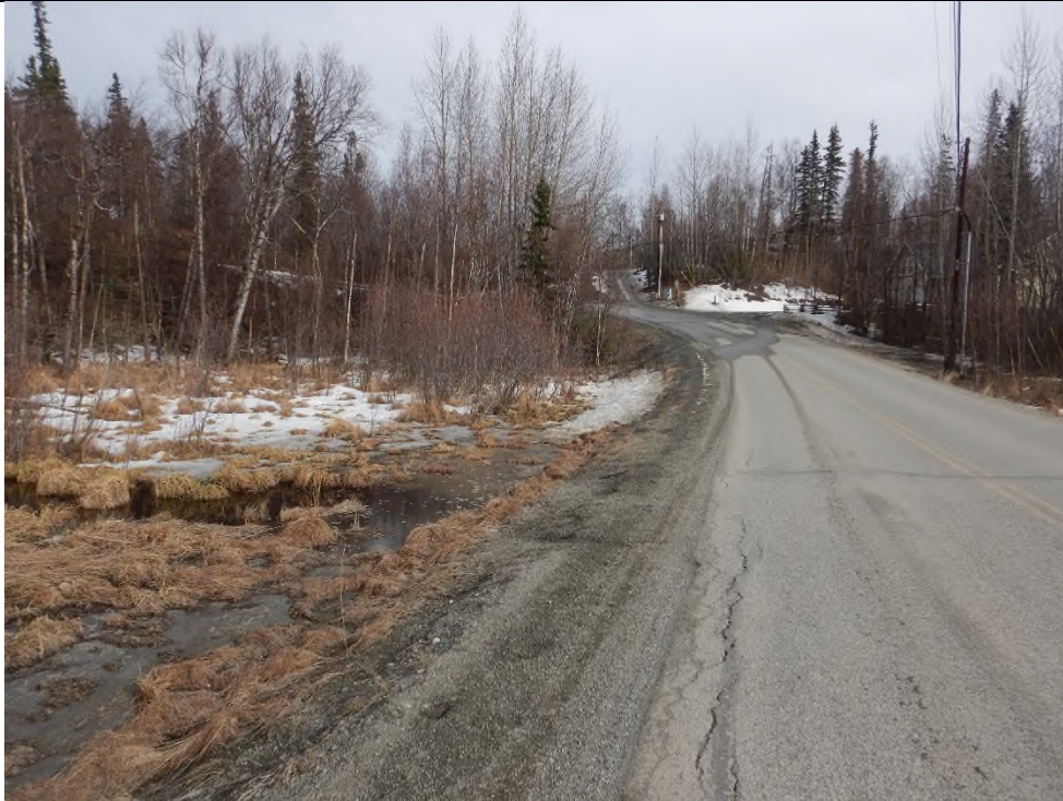
Sediment contamination at sink/channel, north of side of Seagull, east of North 49th State Street.
