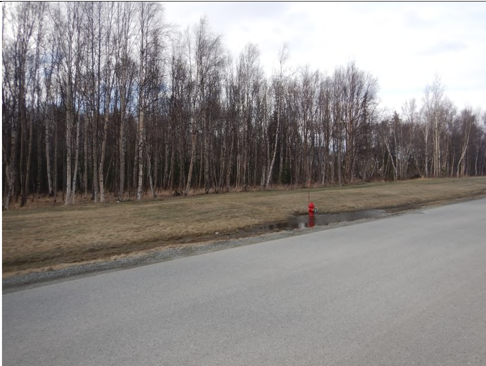
Ponded water at fire hydrant along Fetlock Drive.
