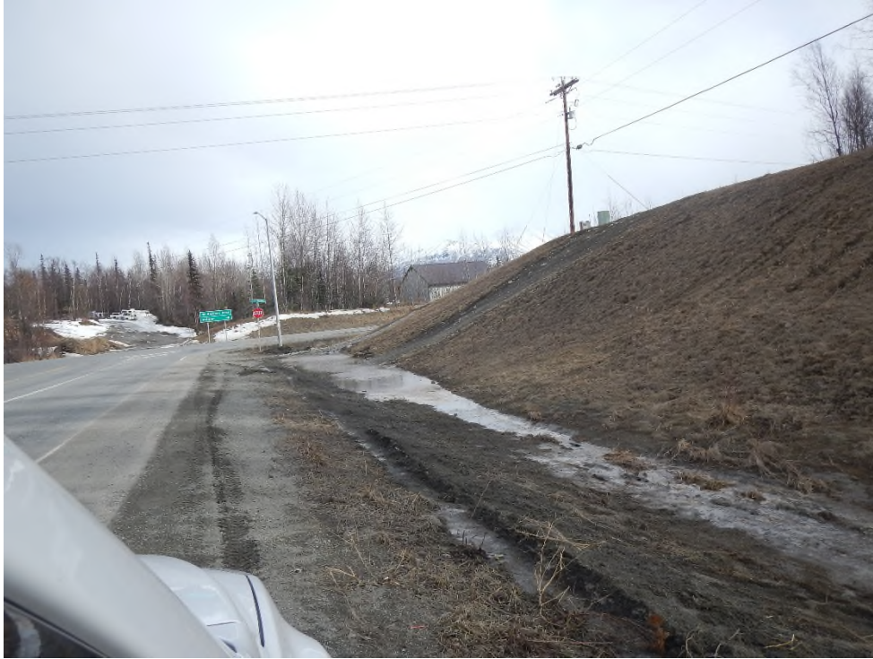
Looking east from Trunk Road toward Palmer-Fishhook Road.
