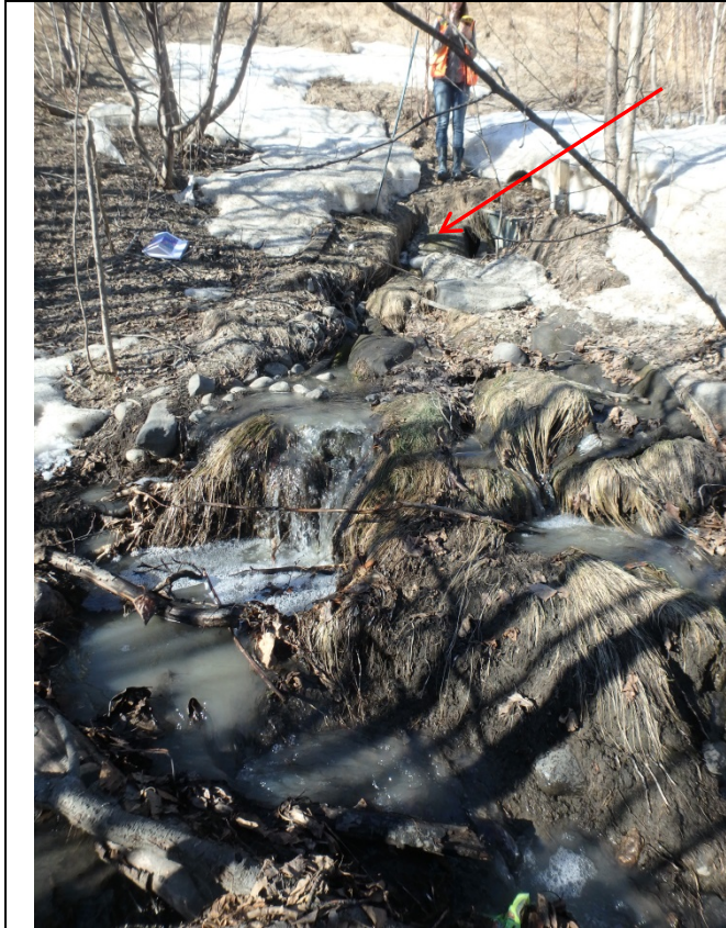
24-inch culvert outlet (draped in geotextile)
