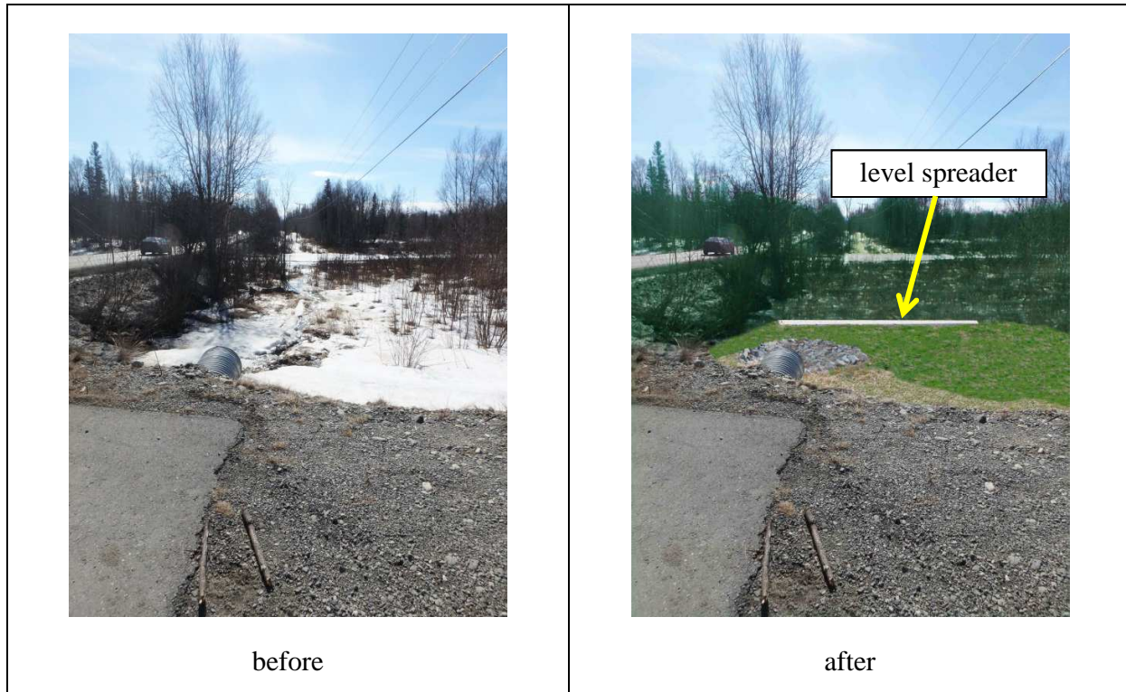
Figure 8: Flow Spreader Facility Concept
