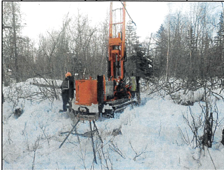
Figure 3: CME-55 Drilling Rig on Proposed Lot 2B (Undeveloped Area)
