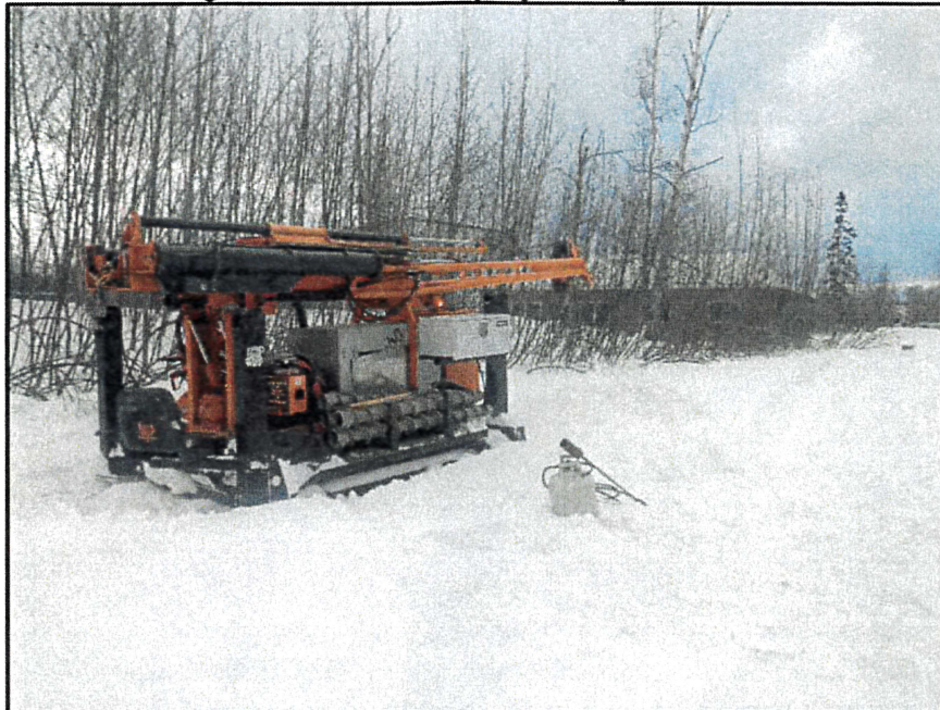
Figure 1: CME-55 Drilling Rig on Proposed Lot 2A
