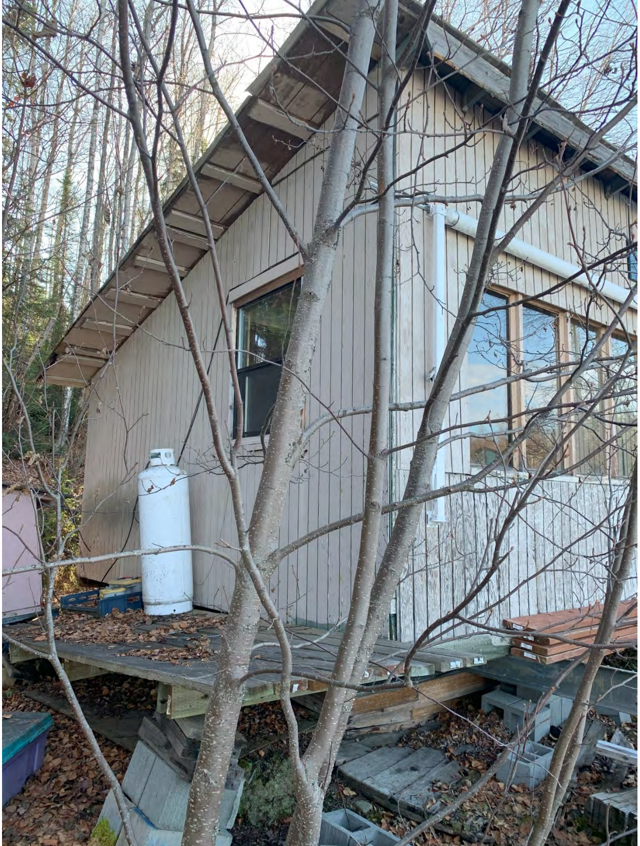
Pointing east. Showing the north and west sides of the cabin.
