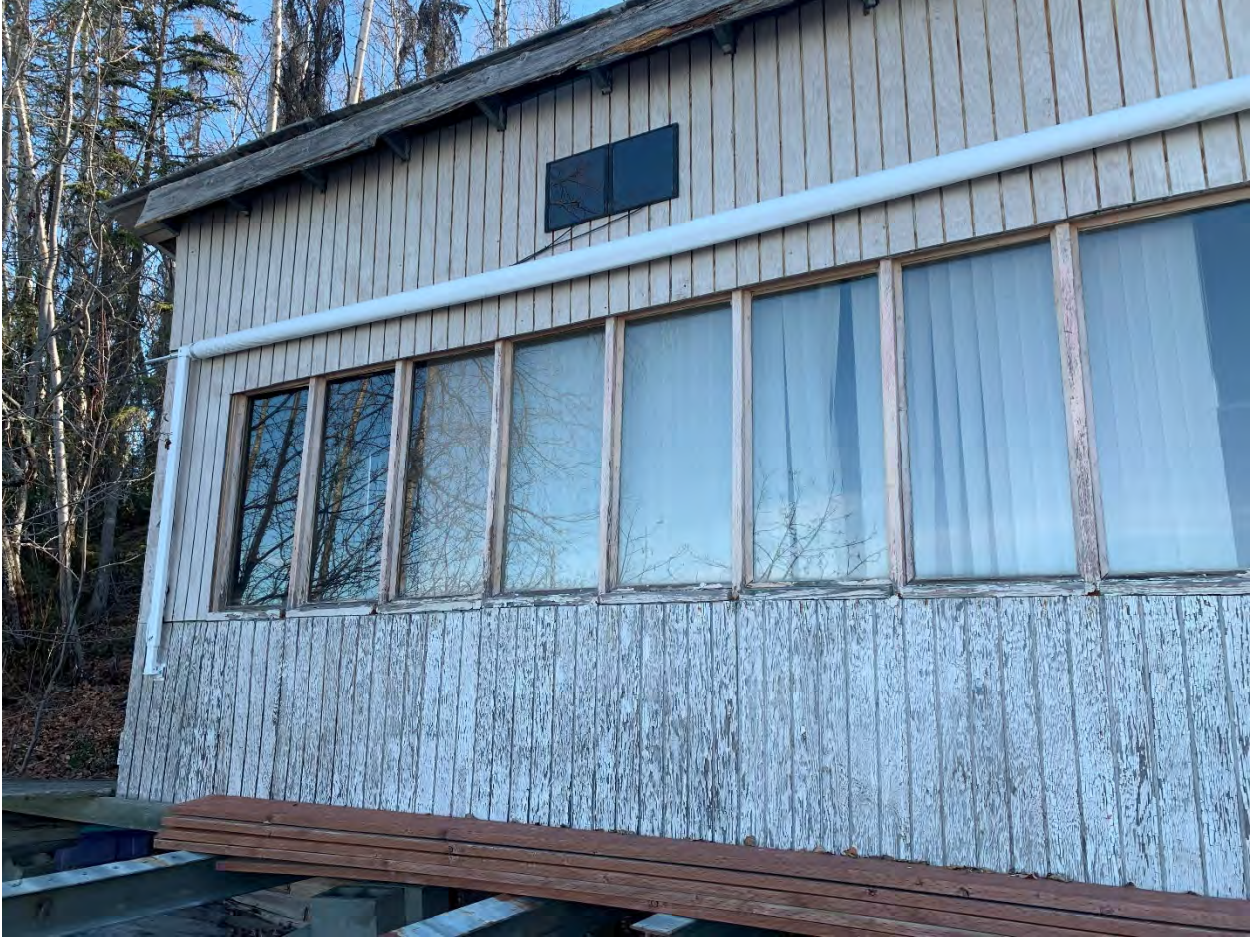
Pointing northeast. Showing the west side of the cabin.
