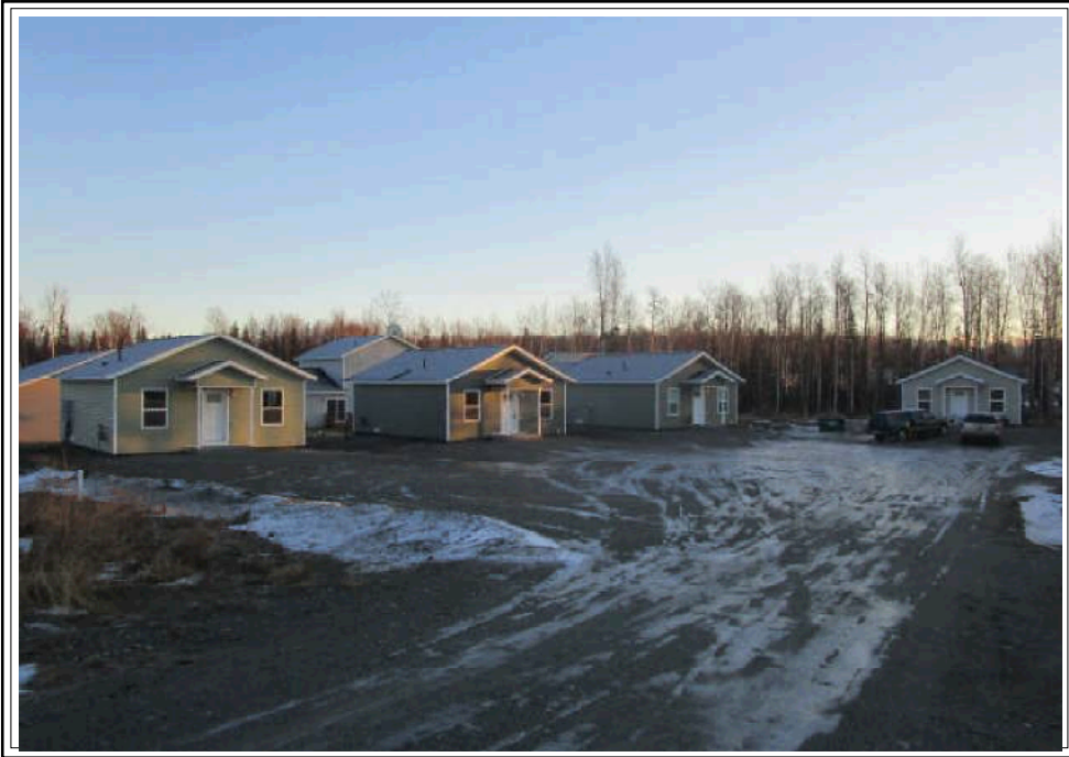
FRONT VIEW OF SUBJECT PROPERTY
