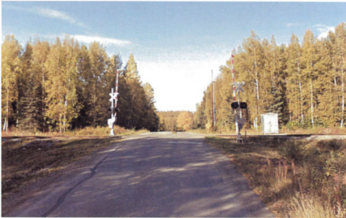
Figure 14. Cheri Lake Drive at-grade Railroad Crossing
