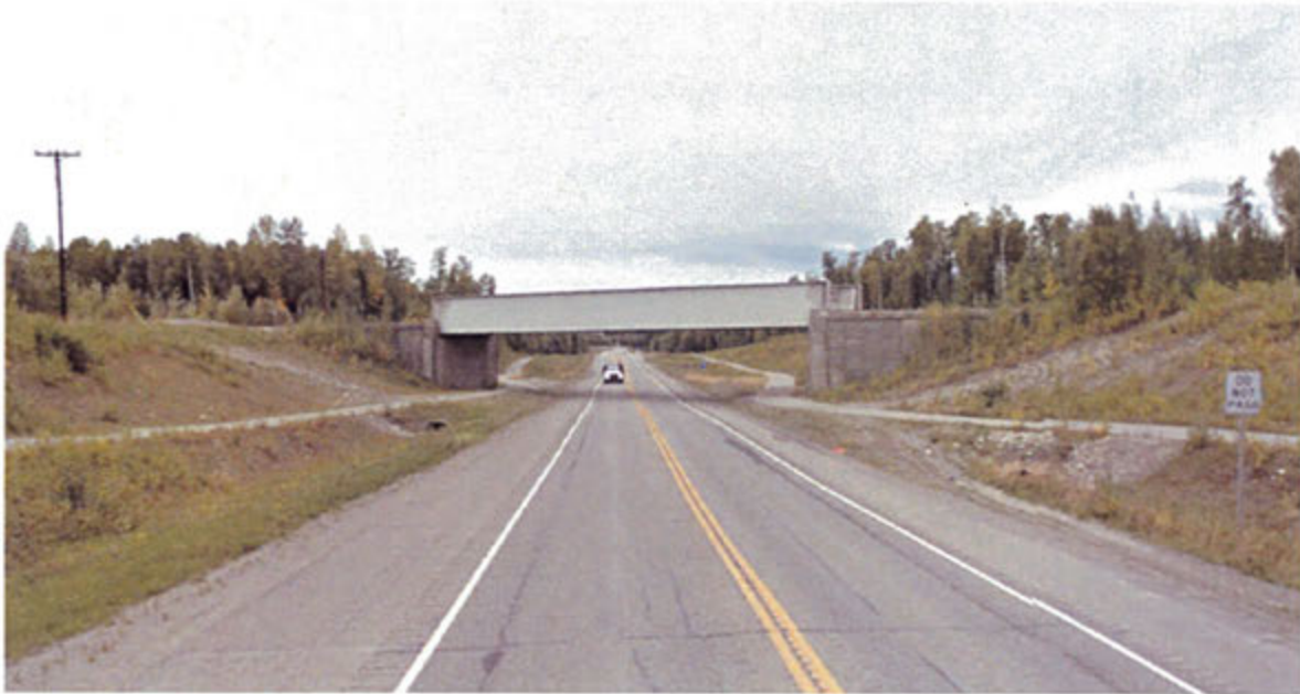
Figure 13. Alaska Railroad Separated Grade Crossing of the Parks Highway
