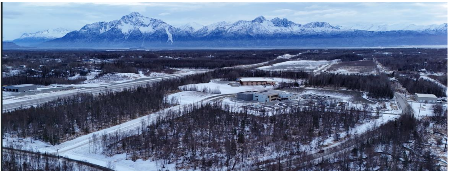
Above photo: Mat-Su Central School as of December 23, 2024
