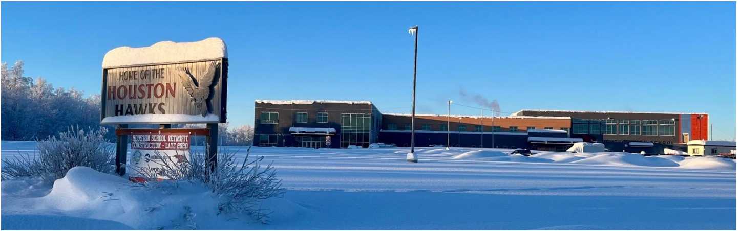
Above Photo: Houston High School Exterior December 2022
