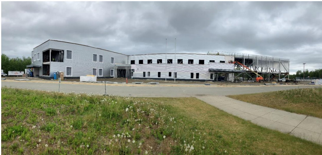
Above photo: Houston High School exterior siding installation
