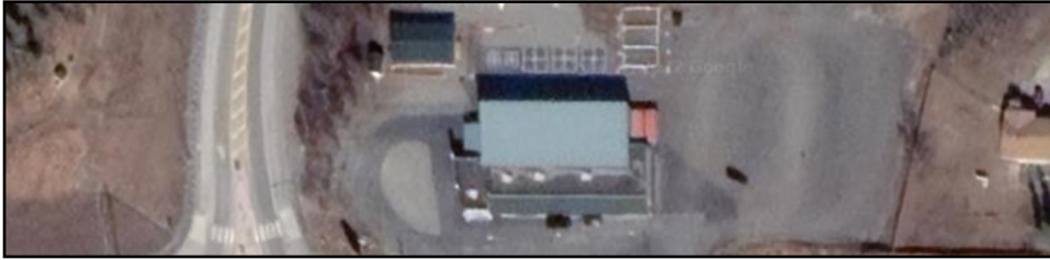
Figure 307. Aerial Photo of Twindly Bridge Charter School.
