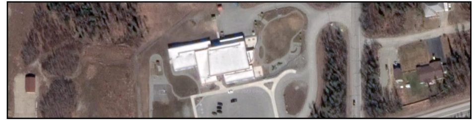
Figure 286. Aerial Photo of Mat-Su Day School.
