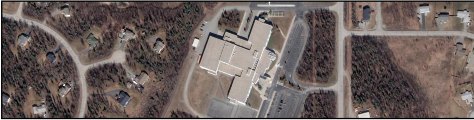
Figure 234. Aerial Photo of Teeland Middle School.
