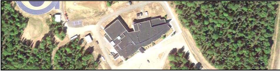
Figure 264. Aerial Photo of Susitna Valley High School.
