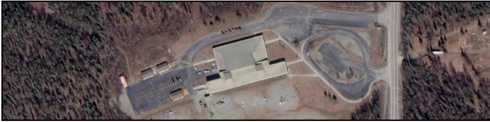
Figure 222. Aerial Photo of Tanaina Elementary School.
