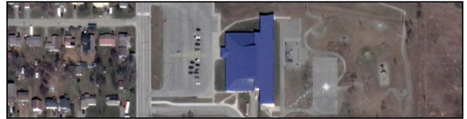
Figure 214. Aerial Photo of Sherrod Elementary School.
