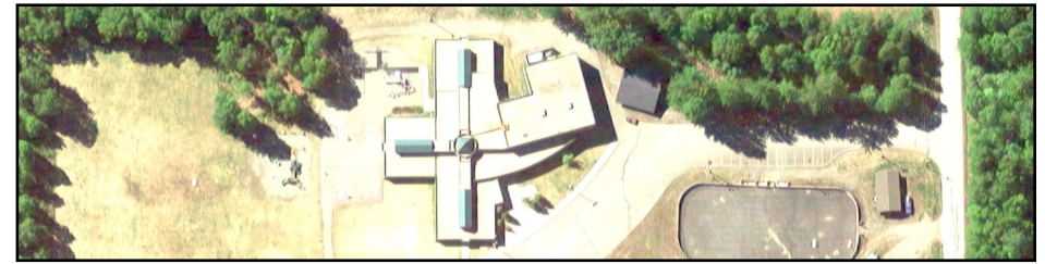
Figure 268. Aerial Photo of Talkeetna Elementary School.
