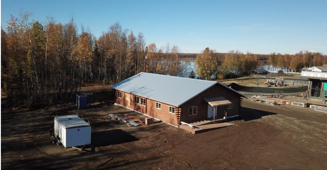
Above photo: Aerial photo of cabin under construction in September 2021
