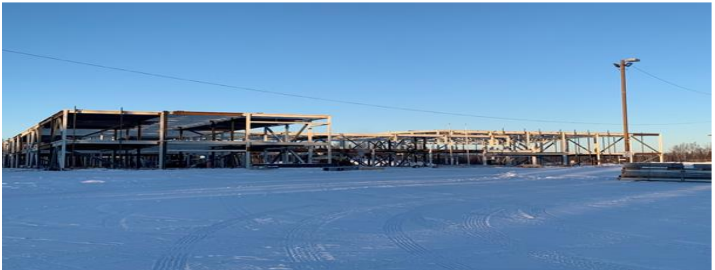
Above photo: Houston High School structural steel complete
