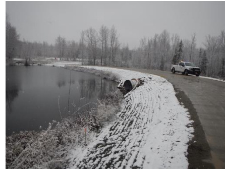
Above photo: Cloudy Lake Outfall After
