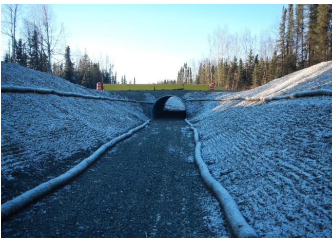
Above photo: Completed trail crossing under Burma Road
