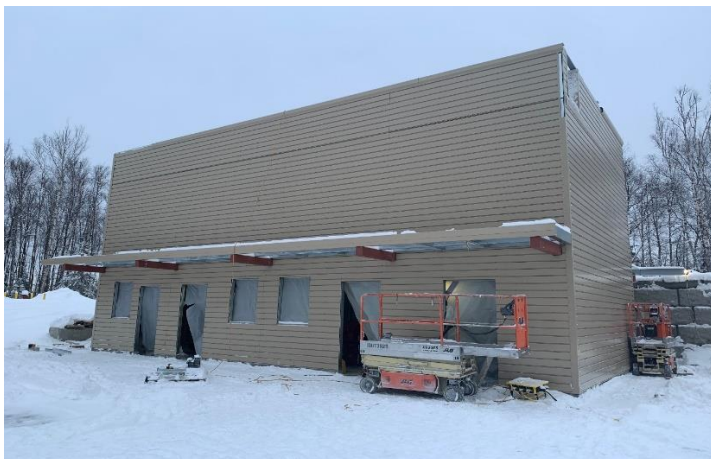
Above photo: 6-2 New Training Tower
