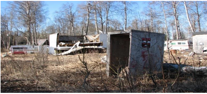
Above photo: before the junk and trash cleanup
