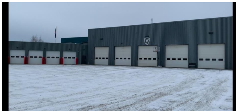
Above photo: New Bays at Station 6-1
