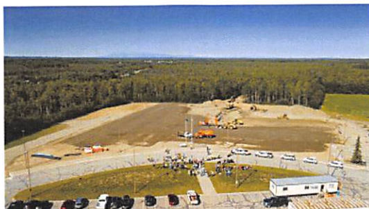
Above Photo: Houston High School Groundbreaking
