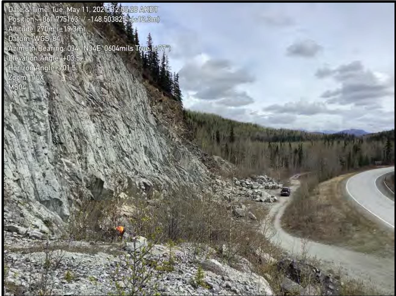
Figure 6. Inactive quarry site adjacent to MSB parcels.
