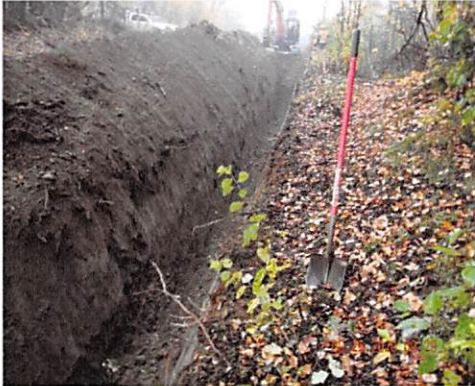
Above Photo: Trenching
