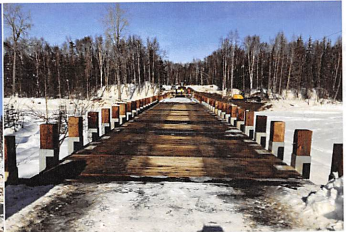
Above Photo: Shirley Towne Bridge re-decking work.
