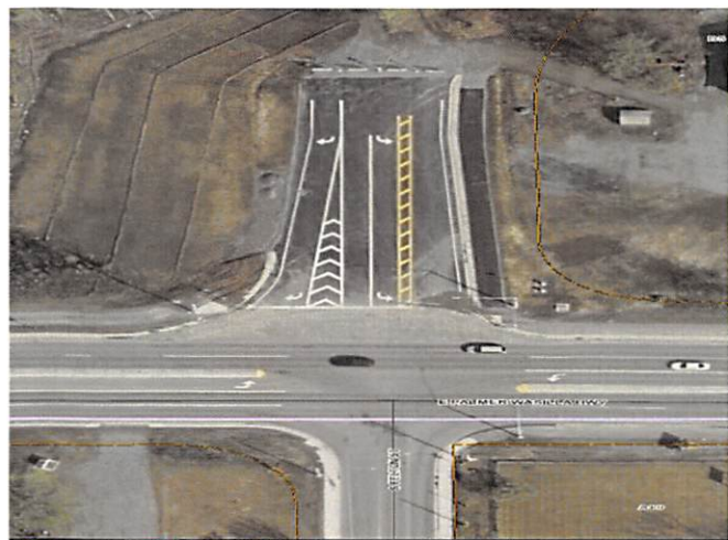
Above Photo: Felton Street approach constructed by ADOT&PF
