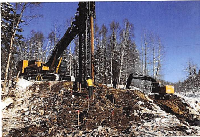
Above Photo: Shirley Towne Bridge Reconstruction
