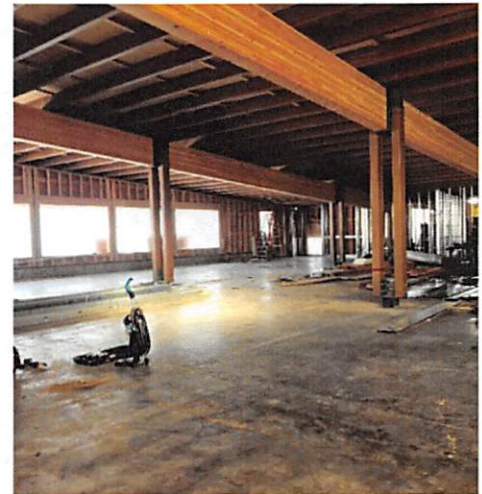
Above photo: Willow Library under construction
