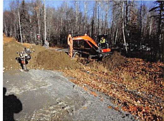
Above Photo: Installing a Telecom Road Crossing
