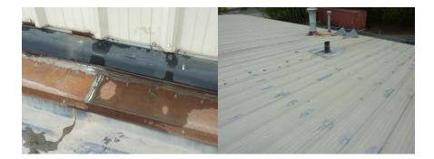
These field repairs were completed with mastics and sealants, so even these repairs would be considered temporary in nature. This is an exposed fastener roof, and sealant has been placed at almost every fastener. This is a point of failure for this type of roof system since with expansion and contraction of the roof itself, it will slowly expand the fastener hole, allowing water to migrate into the facility.
