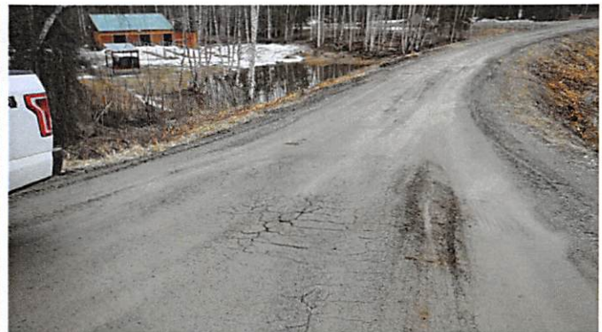
Above Photo: Carillon Road Upgrade Project
