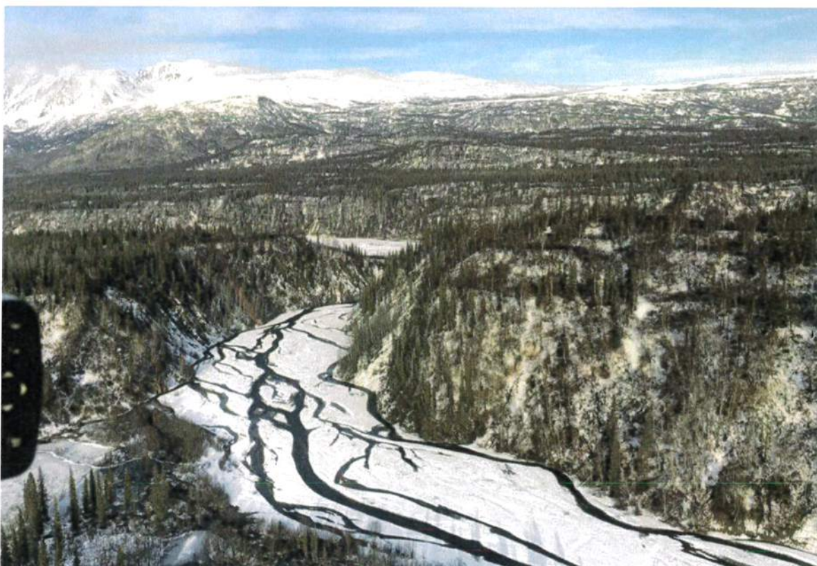
Figure 10: Old Man Creek (looking downstream). Note the steep canyon where the proposed bridge crossing would be located. This bridge would be approximately 1,000 feet long.
