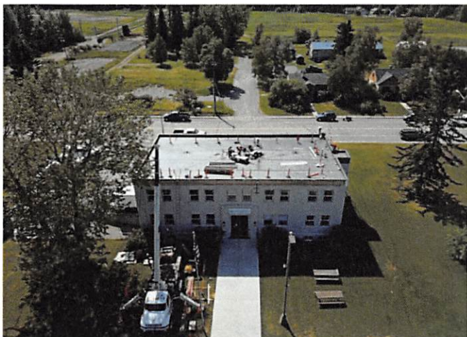
Above: Fireweed Building Roof Repair
