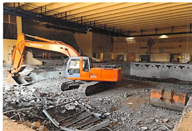
Palmer Pool Demolition
