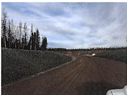
Left: Embankment construction nearing completion
