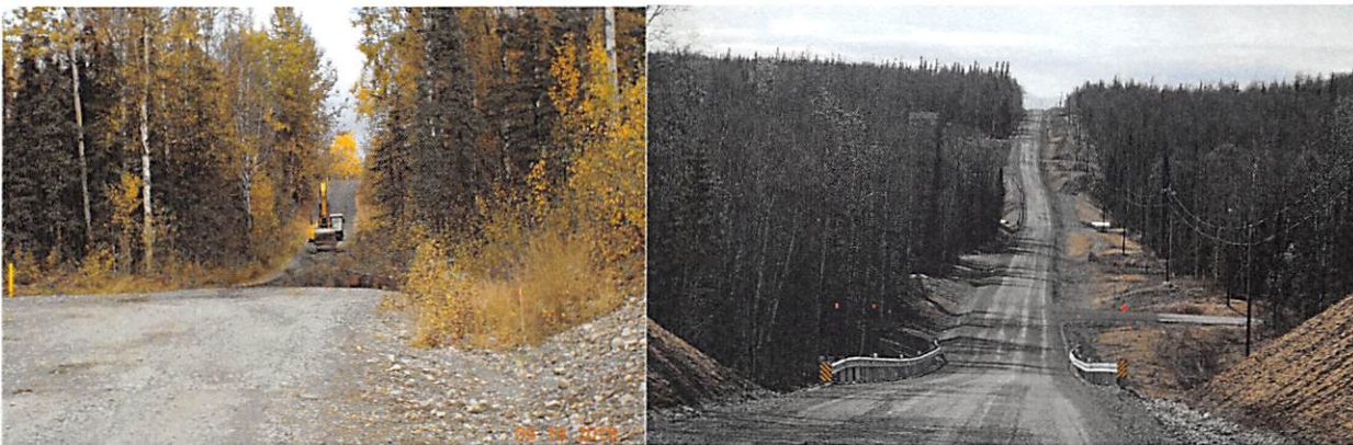
Left: Foothills project, before
