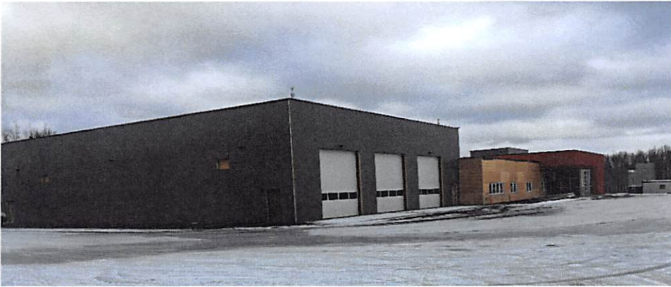
Left: Station 6-2 Construction in progress
