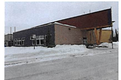
Siding being installed
