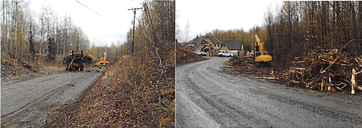
Left and Right: Clearing improvements, Shaw's Tri-Lakes Subdivision
