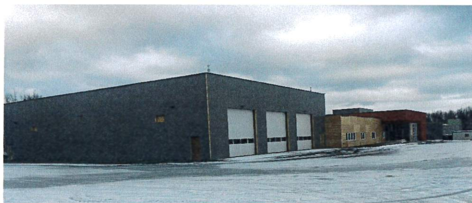
Left: Station 6-2 Construction in progress
