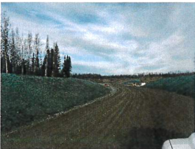
Left: Embankment construction nearing completion
