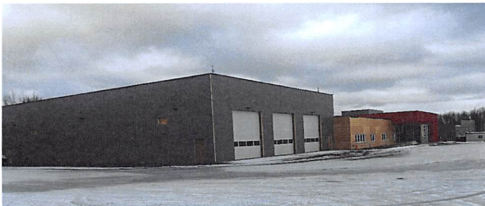
Above: Station 6-2 Construction in progress
