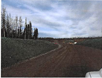
Left: Embankment construction nearing completion
