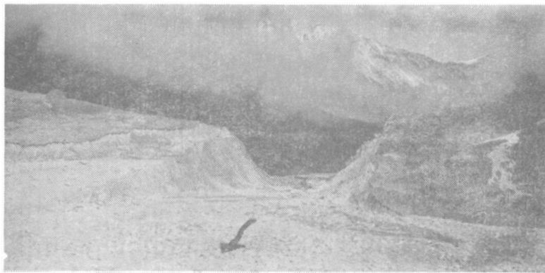
Figure 6.--Breach in embankment of unnamed lake on tributary to Granite Creek.
