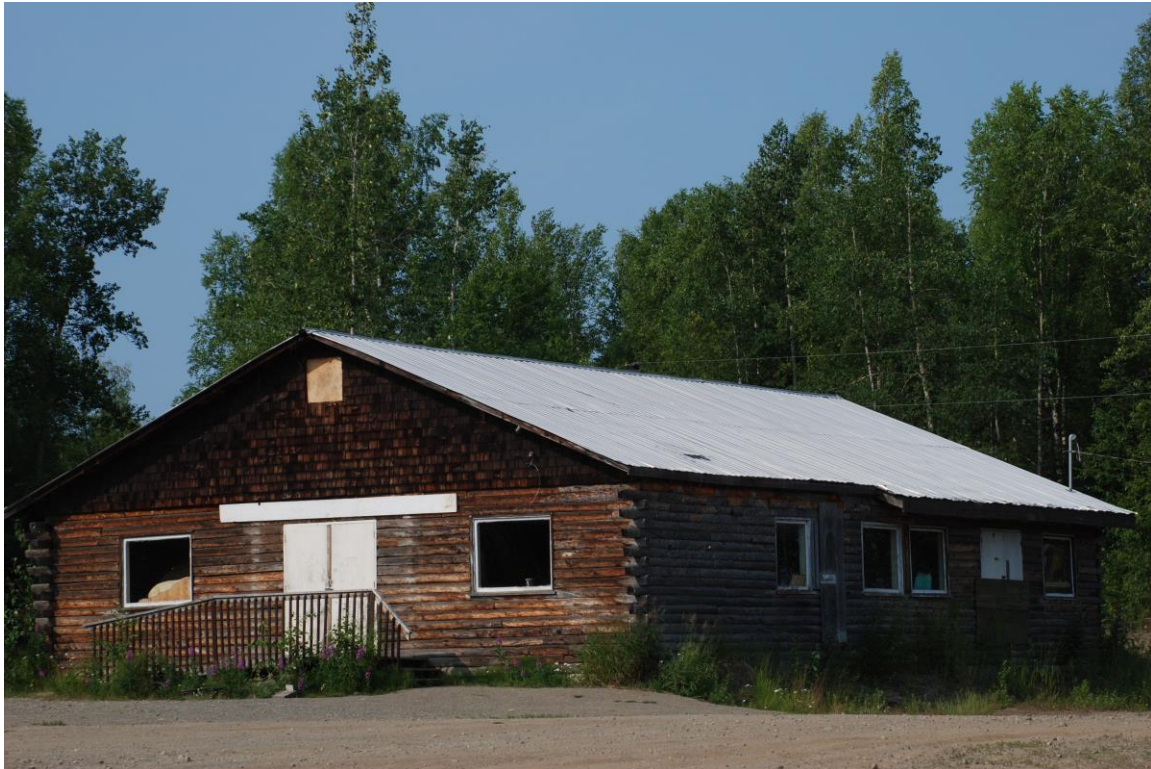
Figure 3.21. Log Building at 69.7 Parks Highway.
