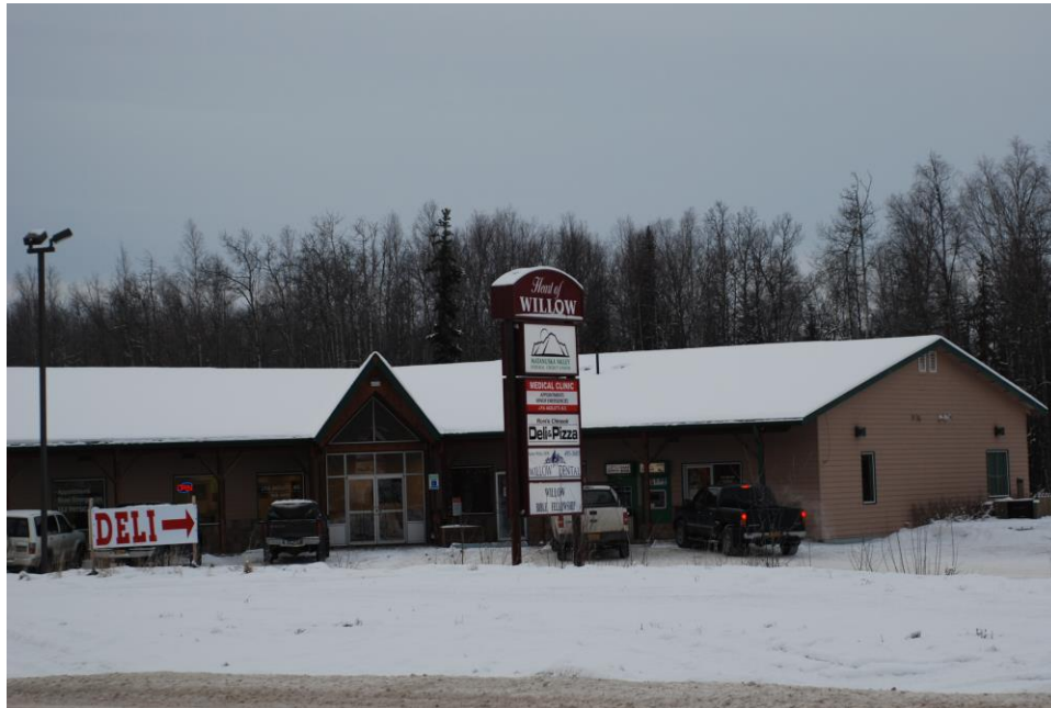
Figure 3.39. Heart of Willow Center – Mile 69.5 Parks Highway.
