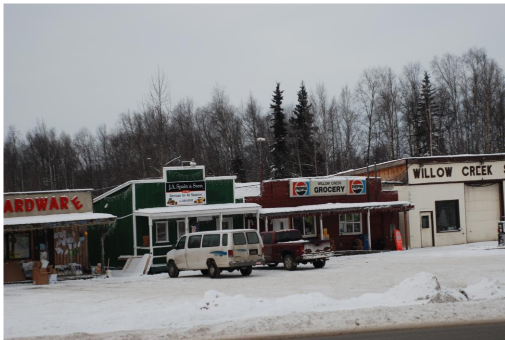
Figure 3.31. J.A. Spain and Sons – 17558 West Parks Highway.
