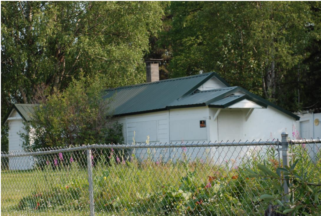
Figure 3.23. Historic Willow Post Office.
