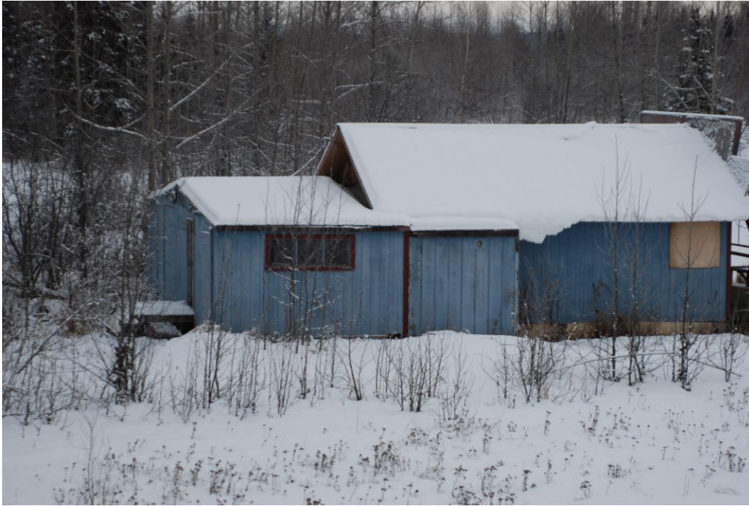
Figure 3.48. Small Building, East Side of Parks Highway - Mile 71.5 Parks Highway.
