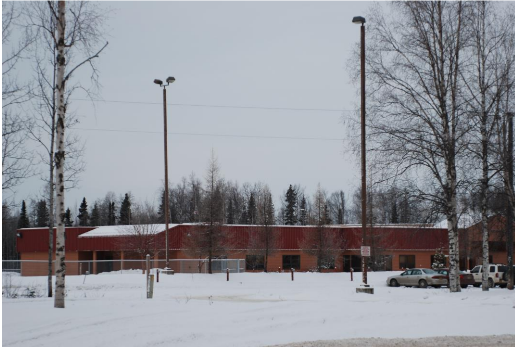
Figure 3.43. Willow School – Mile 69.6 Parks Highway.
