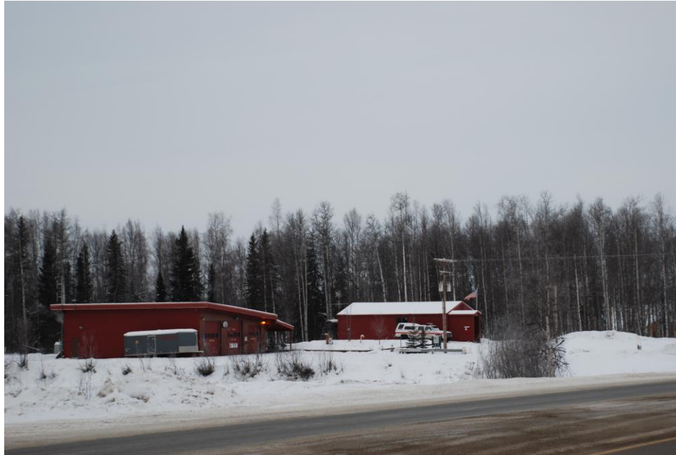
Figure 3.41. Willow Fire Station and Safety Office – Mile 69.9 Parks Highway
