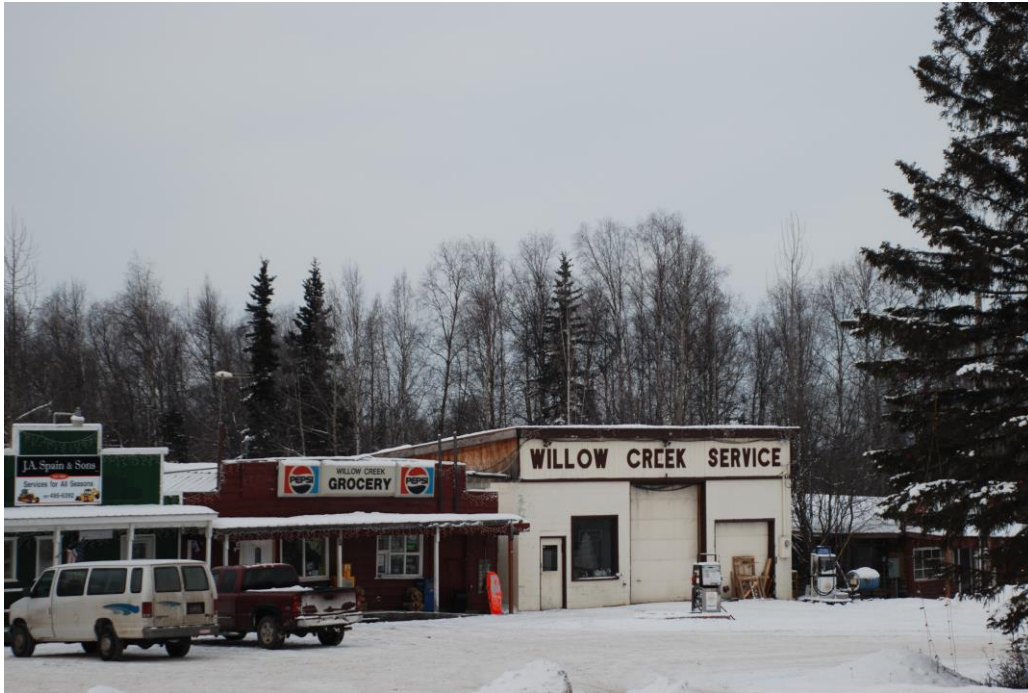
Figure 3.30. Willow Creek Grocery and Willow Creek Service – Mile 69 Parks Highway
