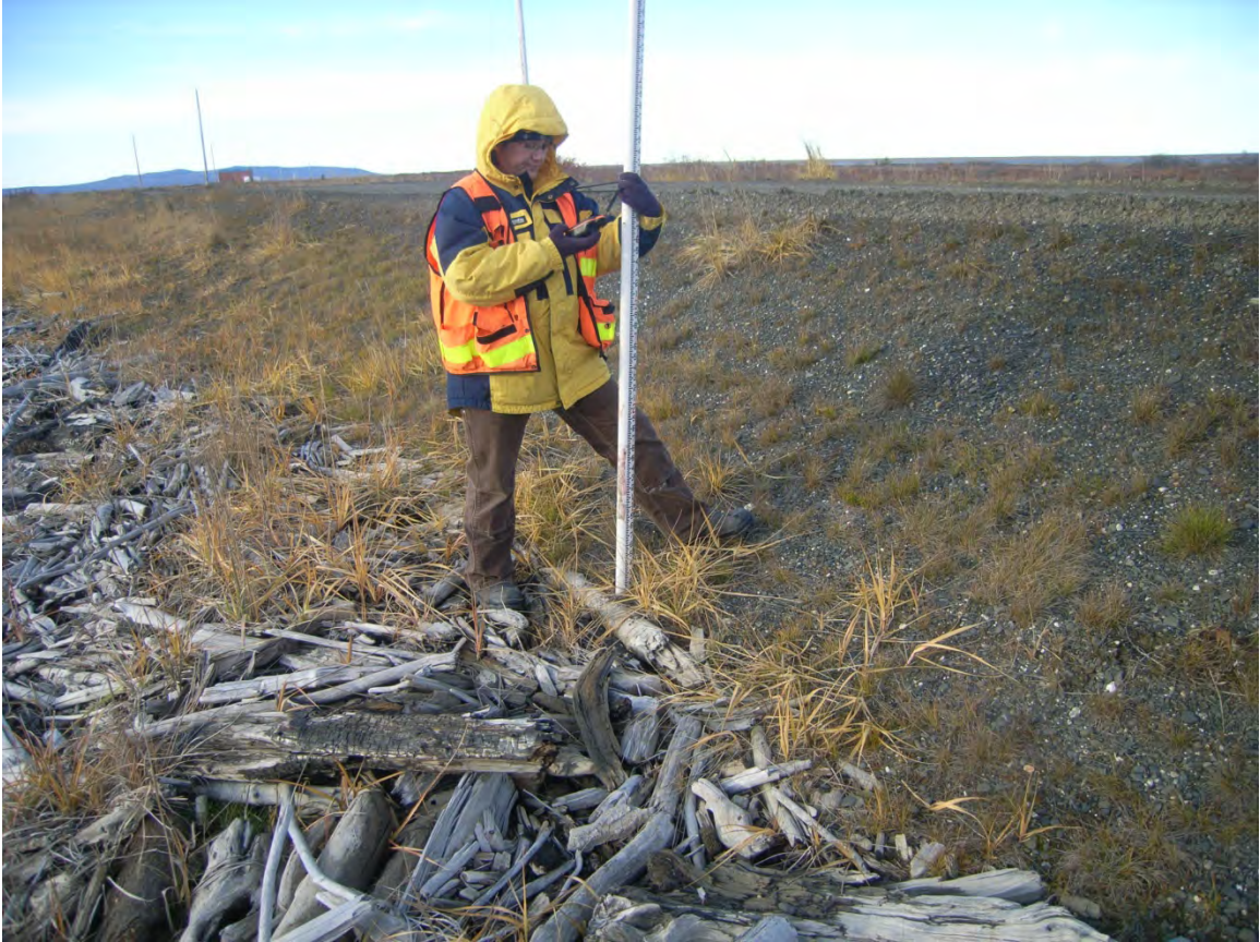
Figure 7: Debris line on road embankment, Poor, Shaktoolik, 2009.
