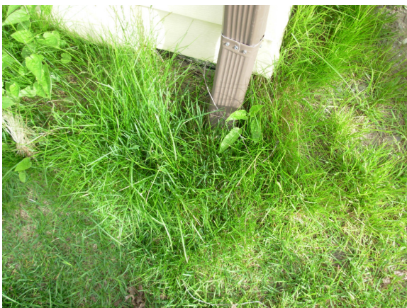
Buried Pipe Entry (buried gutters)
