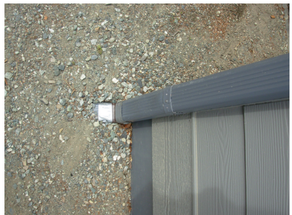
Buried Pipe Entry (buried gutters)
