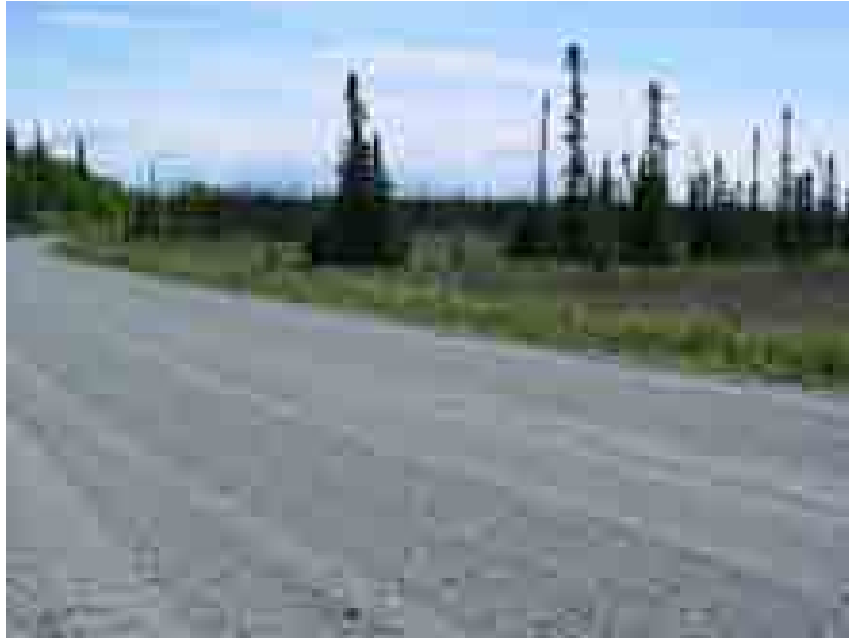
Photo 5: Station East 5, boggy area along Point MacKenzie Road. Looking southeast, road grade approximately 4 feet above marsh elevation.
