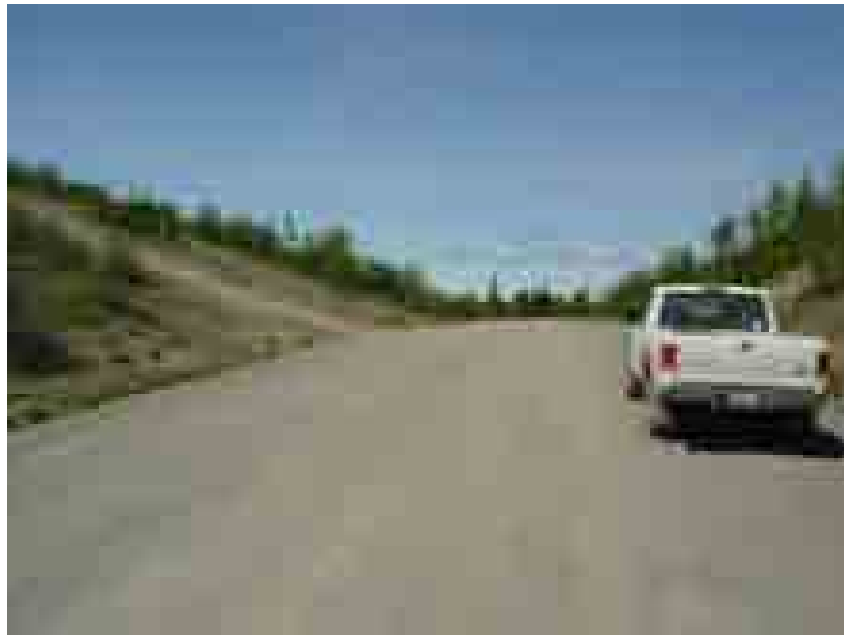
Photo 4: Station East 4, large through cut on West Point MacKenzie Road. Exposed are relatively clean sands and gravels.
