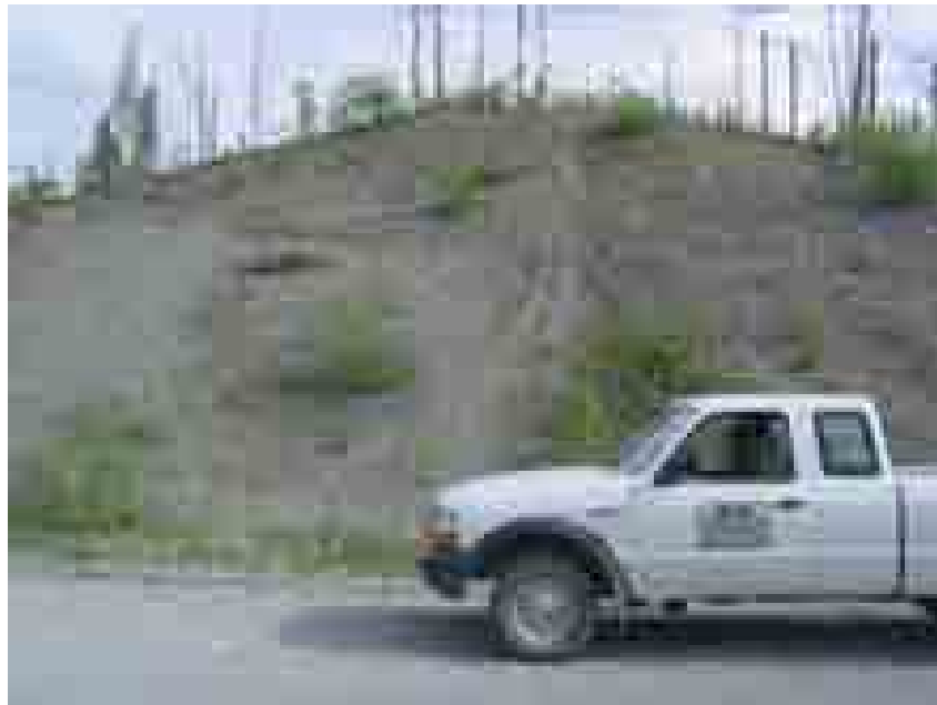
Photo 14: Station East 14, large road cut on south side of West Lakes Road north of Big Lake. Exposed soils consist of clean sands and gravels. These ridges are long narrow features separated by poorly drained marshes and Lakes.
