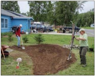
Grooming the topsoil. We created a **berm** on the downslope edge of the rain garden to allow runoff to pond.
