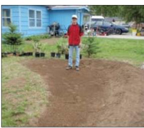
We arranged the plants to follow the layout we sketched. We put the most water-loving plants in the middle of the garden. We placed plants that prefer slightly drier conditions on top of the berm and at the outside edges of the rain garden.
