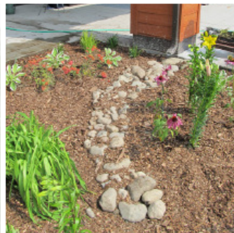
After: Gutter with rock trench to rain garden.
