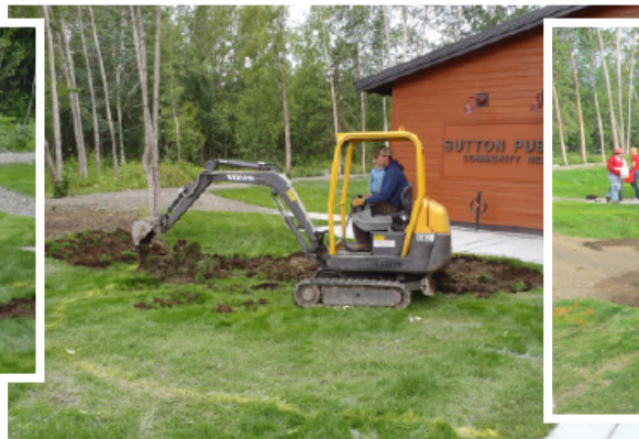
We backfilled with a sand/soil mixture over the gravel for good drainage.
