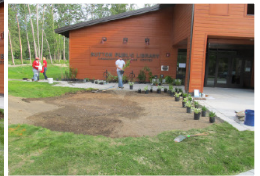
We backfilled with a sand/soil mixture over the gravel for good drainage.
