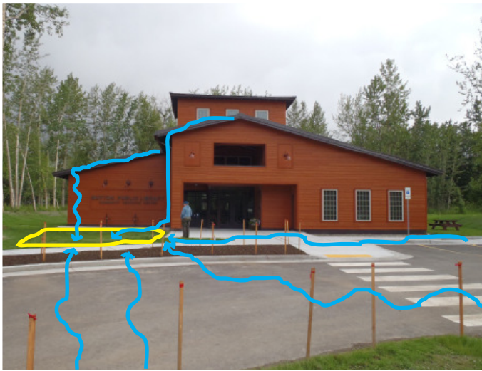
We spray painted an outline for the rain garden after measuring the square footage of stormwater input from the roof, sidewalk, and parking lot.
