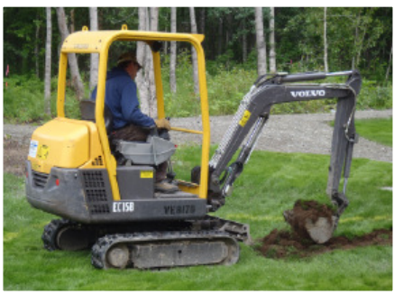
We dug 2-3 feet deep until we hit the gravel layer placed during building construction.
