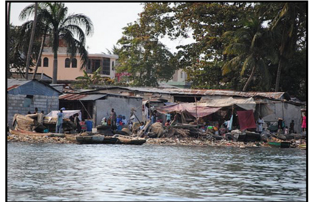
Damage in Port-au-Prince (Photo by Rebekah Runner, courtesy of U.S. Coast Guard)
