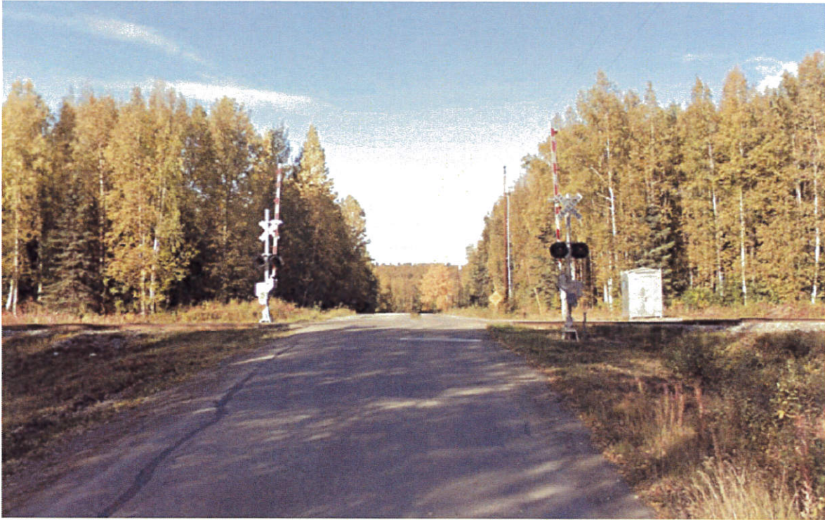
Figure 14. Cheri Lake Drive at-grade Railroad Crossing
