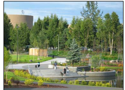
Creation of a multi-purpose retention pond at the Cuddy Family Midtown Park in Anchorage shows an (urban) example of the benefits of “green infrastructure”. This pond was needed to replace wetlands and ponds originally existing in this area. As well as providing (and paying for) a great amenity at the park, this pond captures and infiltrates stormwater from surrounding areas. Building the pond saved hundreds of thousands of dollars that otherwise would have been needed to replace culverts carrying the stormwater runoff from the increasingly developed midtown area to Knik Arm.
