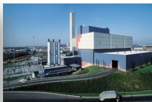
American Ref-Fuel Plant
