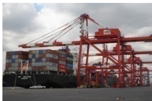
Newark Container Terminal Plant
